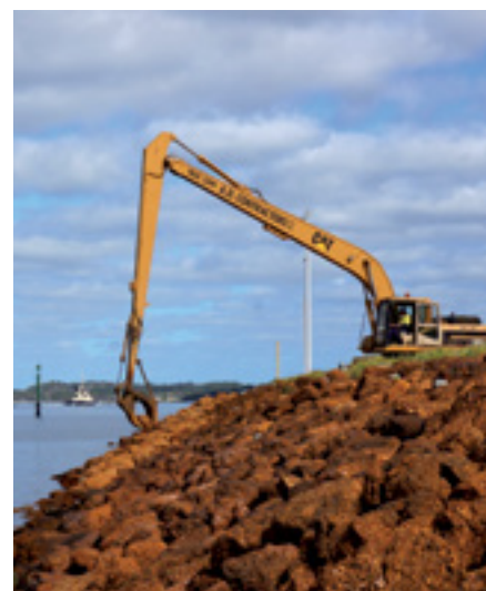
Port of Albany – Repairs to Sea Wall
