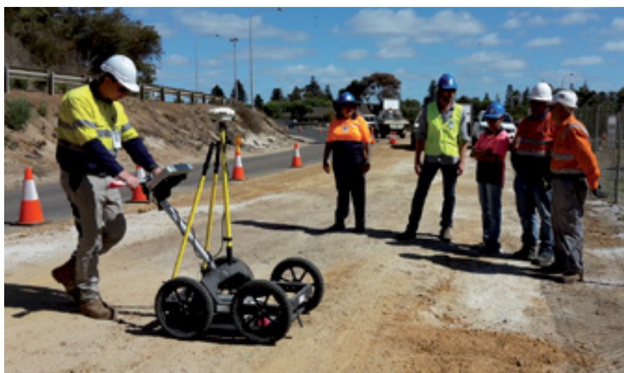
Port of Esperance – Ground Penetrating Radar Survey, Hughes Road
