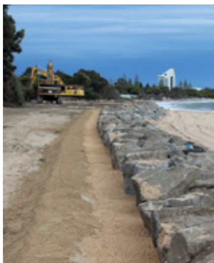
Port of Bunbury - Rock Revetment Wall construction at Point Busaco
