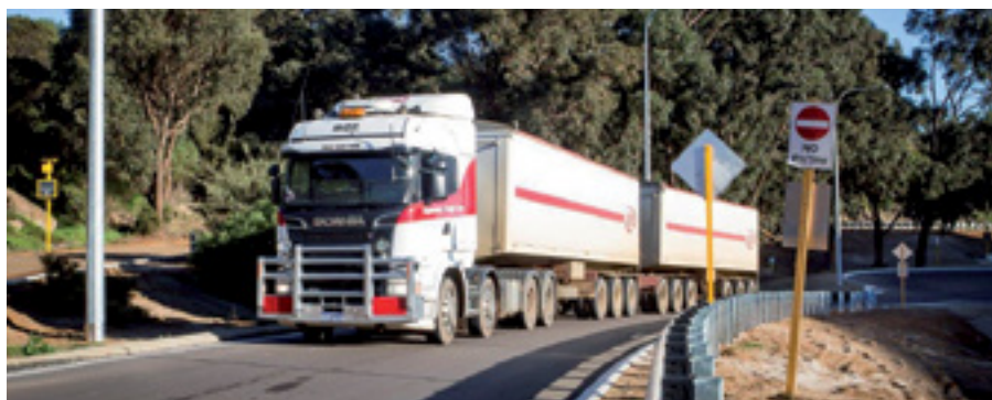
Port of Esperance - Hughes Road upgrade
