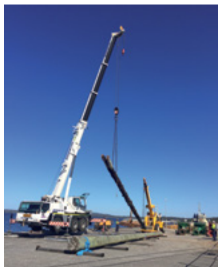
Port of Albany – Timber Fender Replacement Berths 1 and 2
